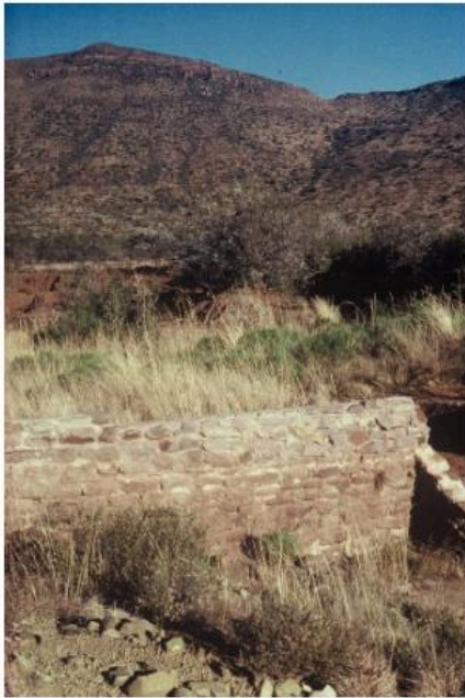
▲ Figure 5.3.2 Check dam to reduce soil loss and water loss
