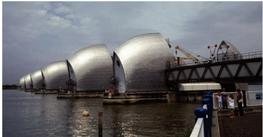
▲ Figure 7.3.1 The Thames Barrier which protects London from tidal flooding. Rising sea levels will mean the Barrier is closed more frequently
