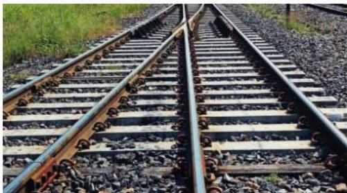
▲ Basalt railway ballast.
