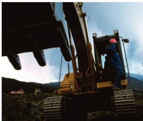
▲ The tracks on the earthmover stop it sinking into the mud.
