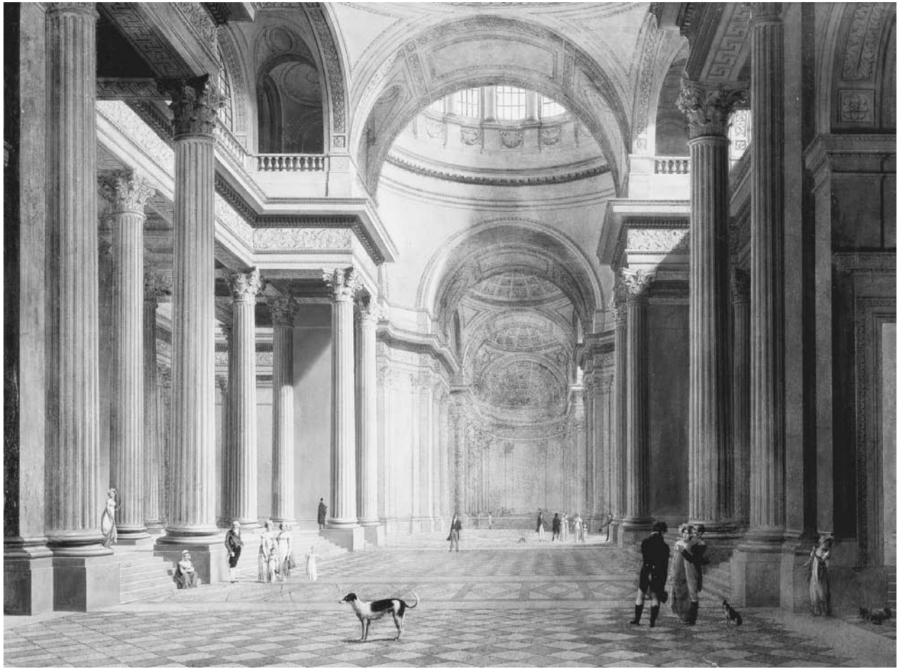
Nineteenth-century drawing of the Panthéon (originally Church of Saint Geneviève), Paris, France. Constructed 1755–1790. During the Age of Enlightenment, attention began to be paid to different methods of structural support, one example being the freestanding columns Jacques-Germain Soufflot used in his design for the Panthéon. © ARCHIVO ICONOGRAFICO, S.A./CORBIS
