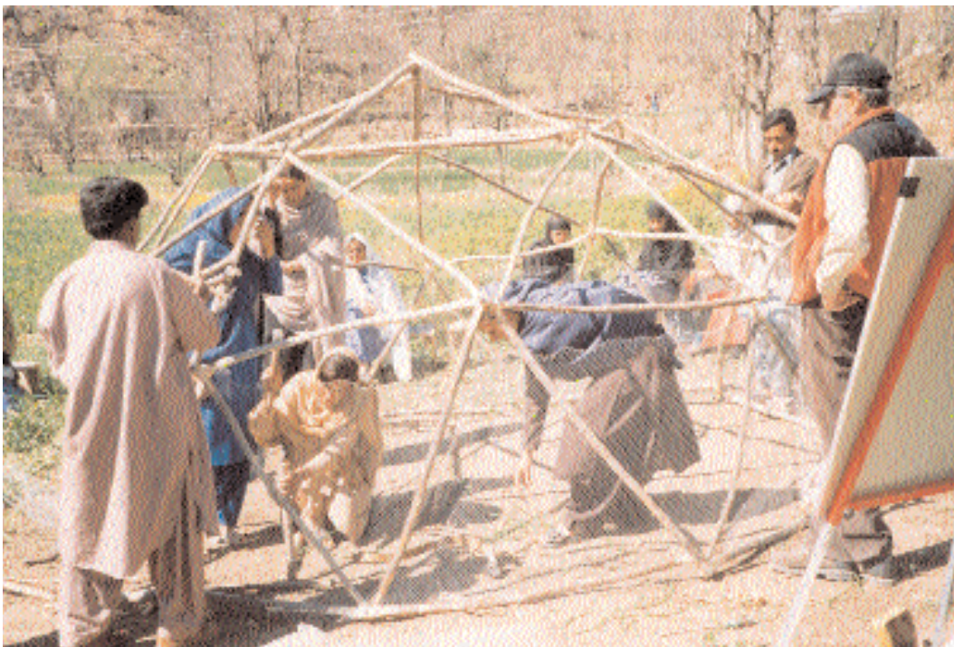
A resource person from an NGO teaches the construction of a multi-purpose dome structure to women farmers and Female Extension Assistants under training at Garhi Dopatta.
