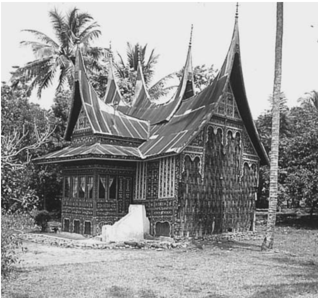
Minangkabau house, with multiple gables covered with carved and painted wood panels and upward arching roof ridges. Sections of the wall are still in progress, later to be covered with carved panels. Courtesy of Andrew Causey. Used by permission.
