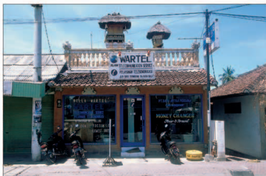
Wartel office providing phone services
