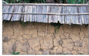
A courtyard wall built of clay and capped with bamboo
