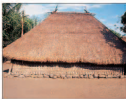
A house in Segenter, constructed from parts of the coconut palm
