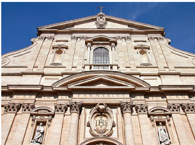
The Counter-Reformation-style facade of Chiesa del Gesù (p81)
