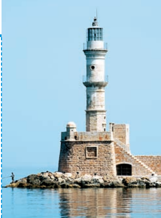
The minaret-style lighthouse.
