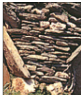
Unmortared wall of schist slabs
