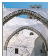
Arched buttresses for earthquake protection
