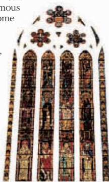
A large window in the south wall
