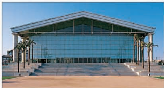
The façade of the modern Teatre Nacional de Catalunya
