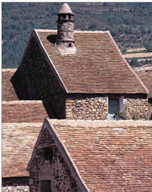
Steep, tiled roofs of Hecho, with a typical pepperpot chimney
