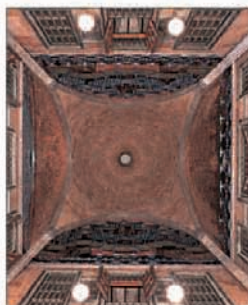
A dramatic cupola covers the central salon, which rises through three floors. It is pierced by small round holes, inspired by Islamic architecture, giving the illusion of stars.
