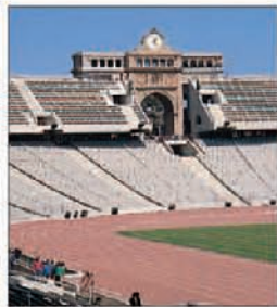
Entrance to the refurbished 1992 Olympic Stadium
