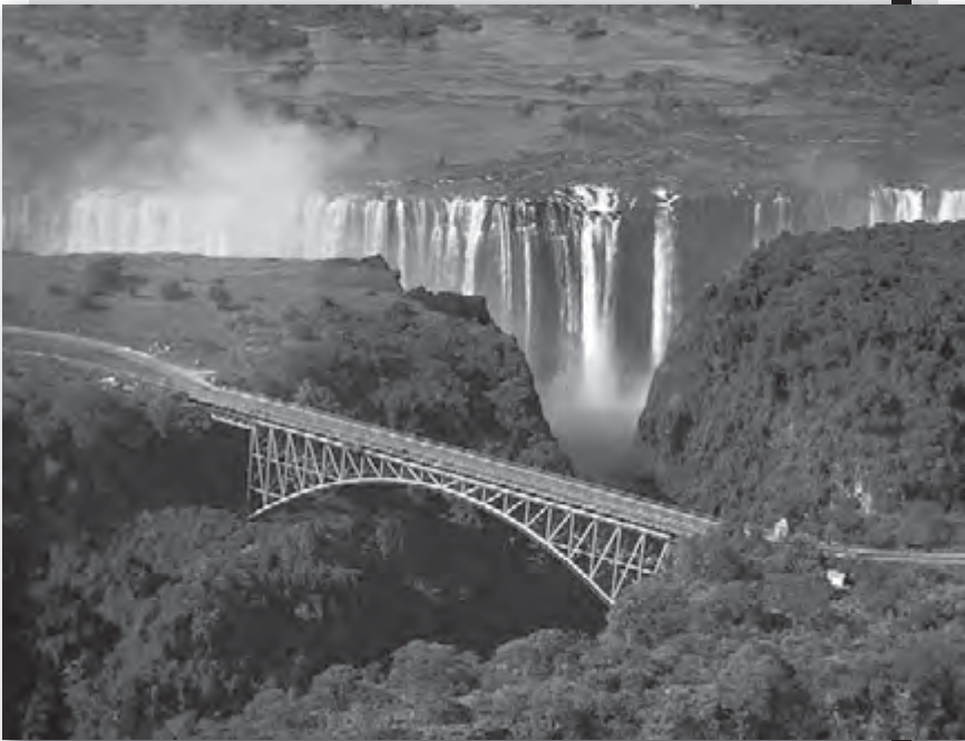
The Victoria Falls Bridge across the Zambezi River, connecting Zambia and Zimbabwe. © Brian A. Vikander/West Light
