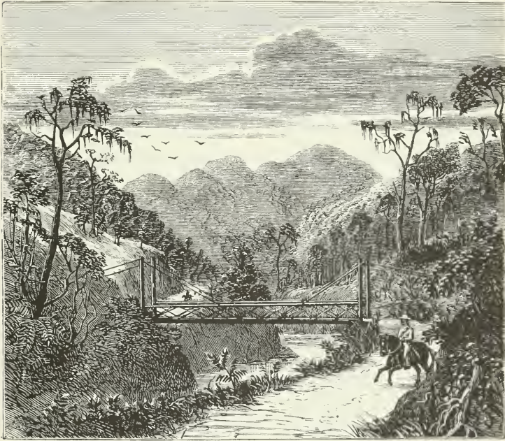
A BRIDGE ON THE MOUNTAIN ROAD TO THE COAST.
