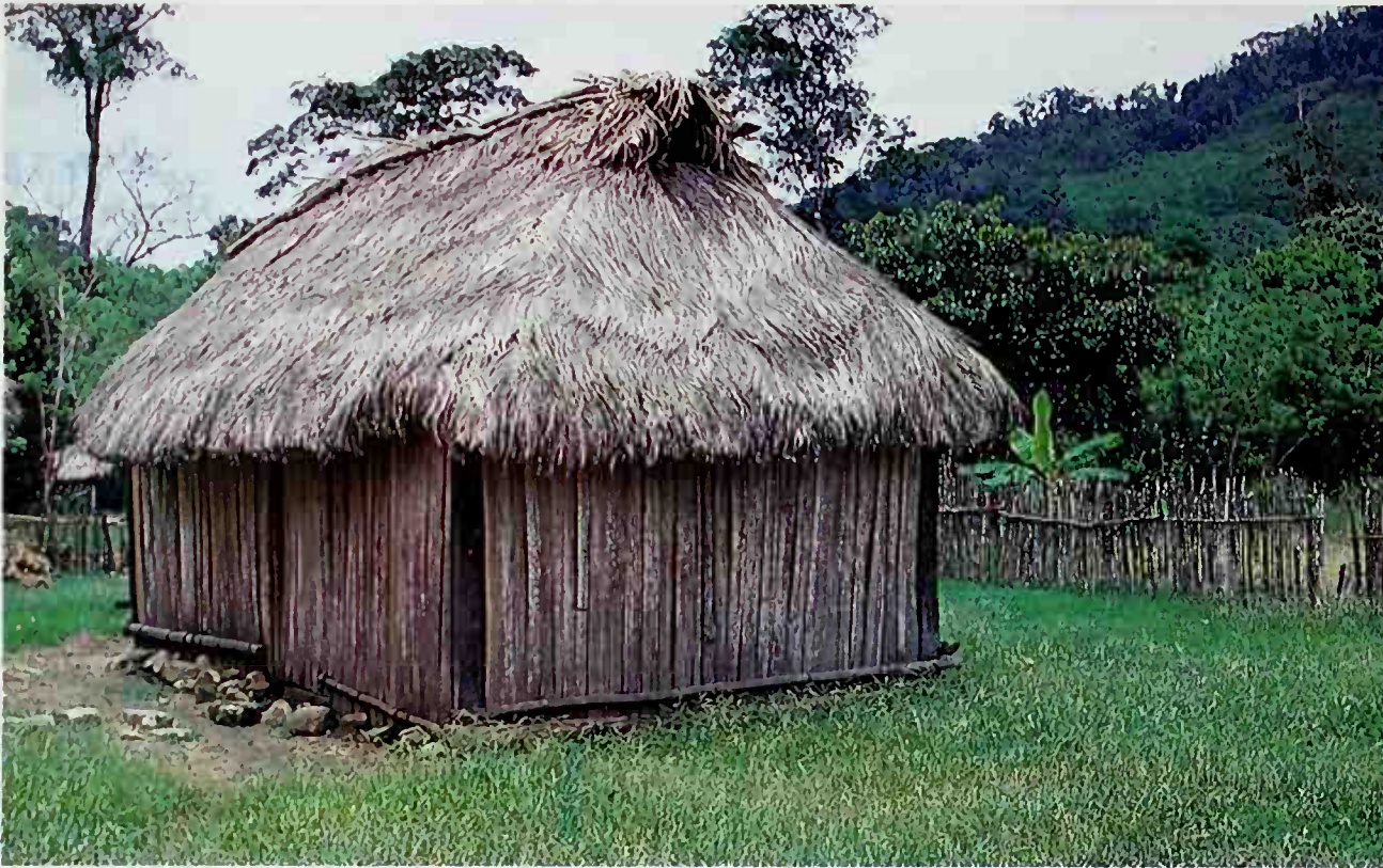
The houses where the common people lived were similar to those which are still used as dwellings for the peasants of the Mayan area. The buildings have walls from wood and straw roofs. The main floor was almost always rectangular, but it could also be apsidal with rounded ends. In this photograph one sees a Tzeltal house in the municipality of Ococingo, Chiapas.
