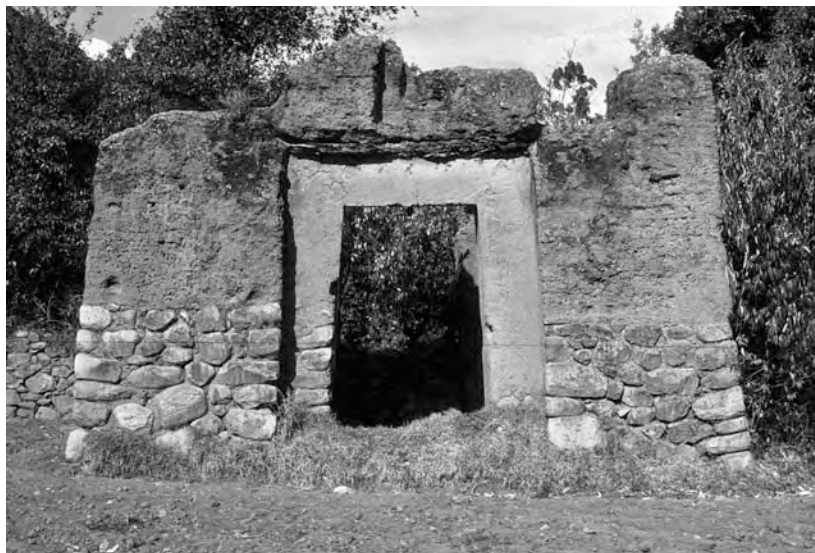
FIGURE 58.1. The remains of Inca buildings in Yucay
