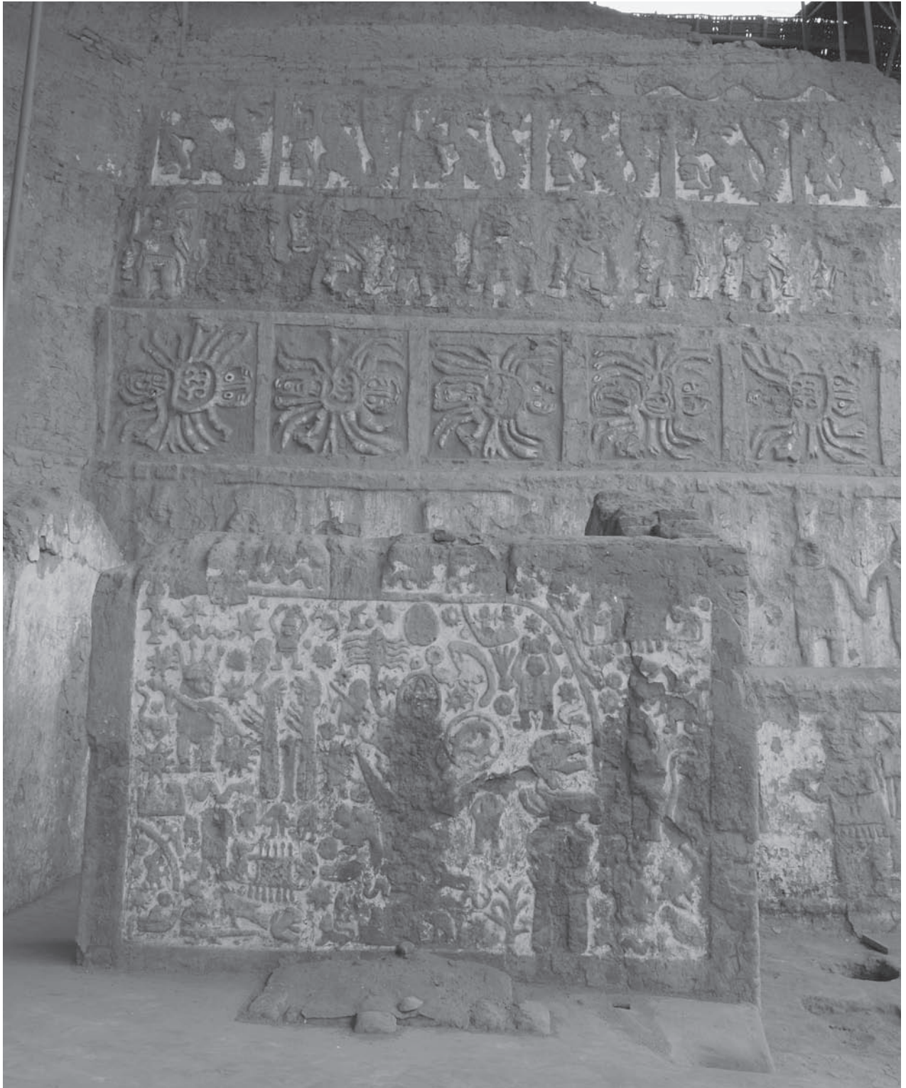
FIGURE 1.17. Huaca de la Luna, detail of north facade mural. Photograph by Steve Bourget.
