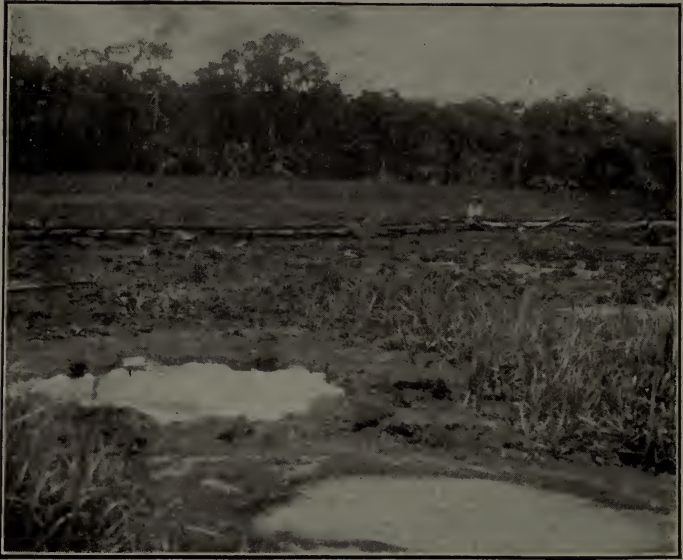
FIG. 47. PITCH LAKE, SHOWING FRESHLY DUG PIT FILLED WITH WATER; AN OLDER PIT FILLED WITH SOFT PITCH, BOTH SURROUNDED BY THE HARD SURFACE PITCH.
