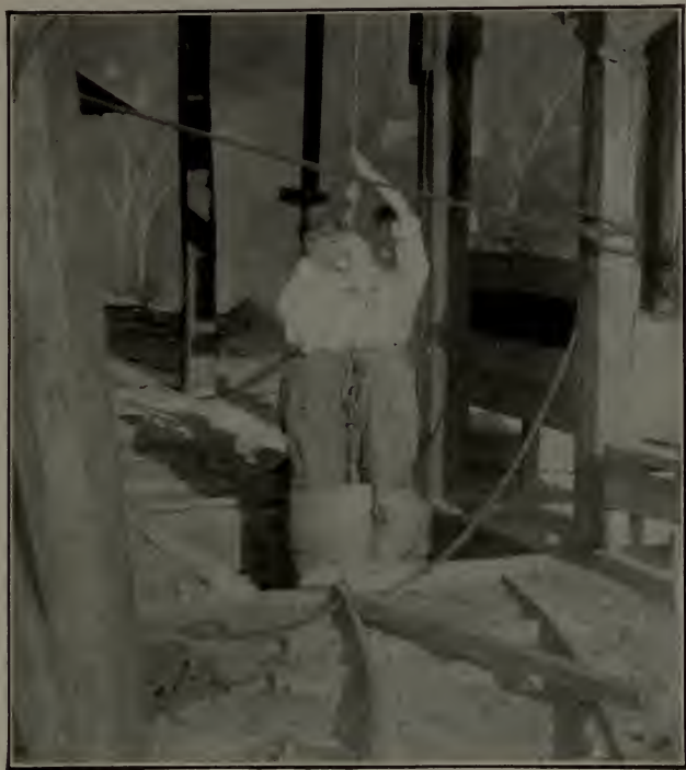
FIG. 125. DESCENDING THE SHAFT.
