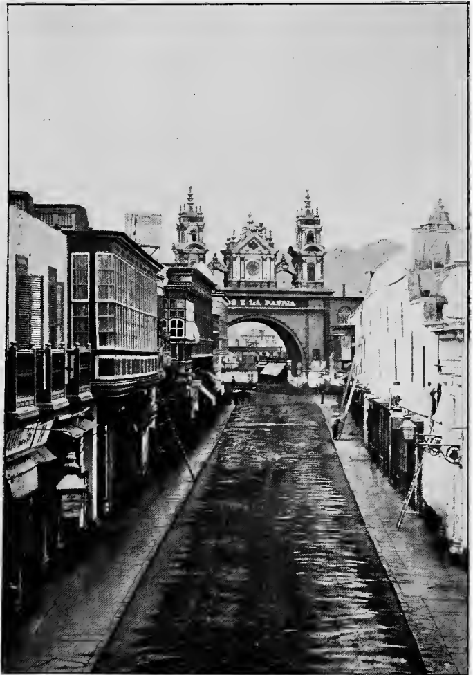
LIMA — Bridge Arch
