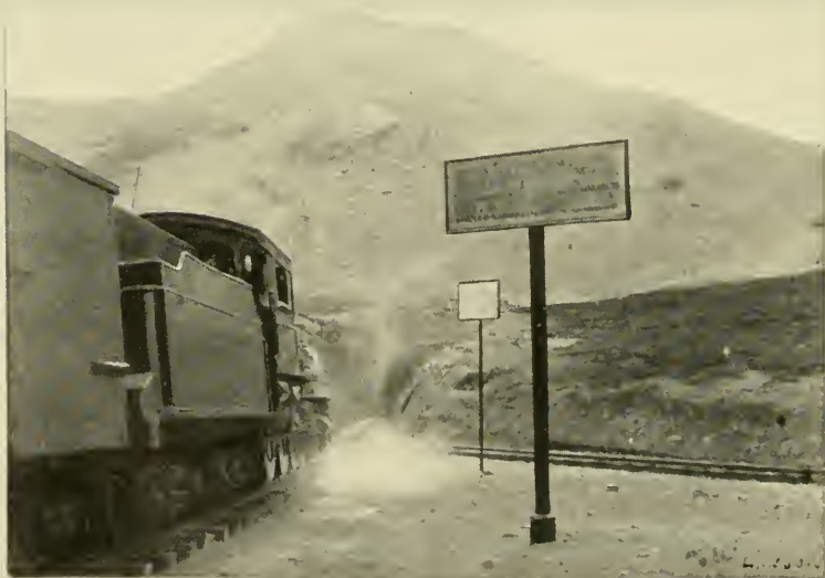
THE HIGHEST POINT OF THE OROYA RAILWAY. The Galera Tunnel.
