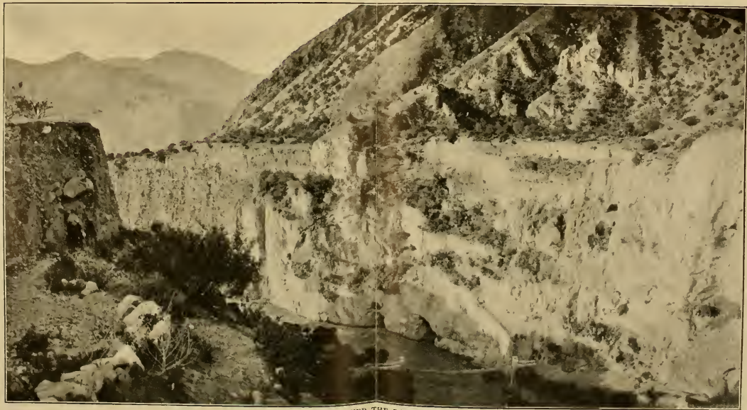
THE BRIDGE OVER THE RIVER PAMPAS
