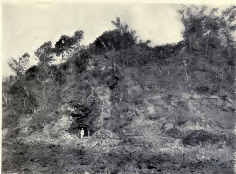
LONGOS MINE, ENTRANCE.
