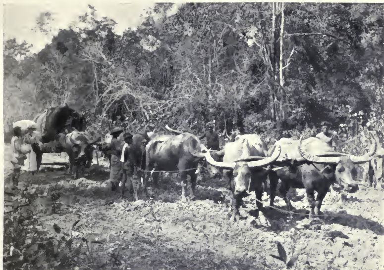
ARRIVAL OF MACHINERY AT KABIN.
