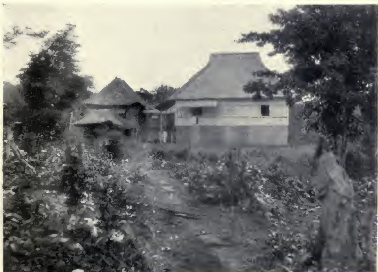
LONGOS MINE, BUNGALOW.
