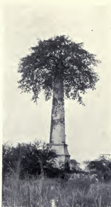
TREE GROWING IN CHIMNEY AT PECHIM.
