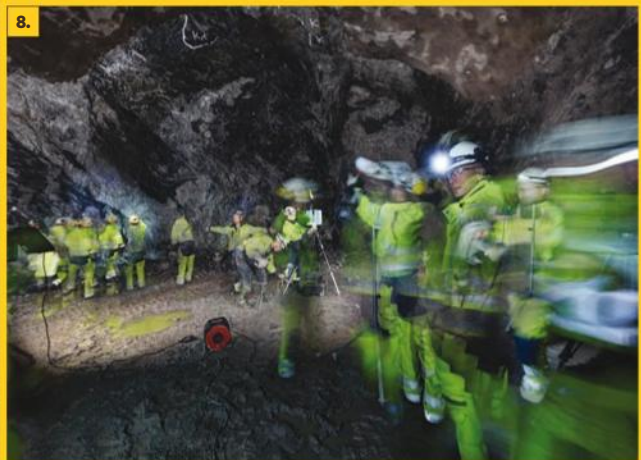
8. Engineers use 3-D scanners to measure the tunnels after drilling and blasting.
