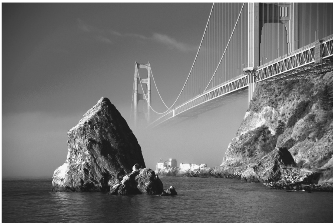
The Golden Gate Bridge. Courtesy of Corbis.
