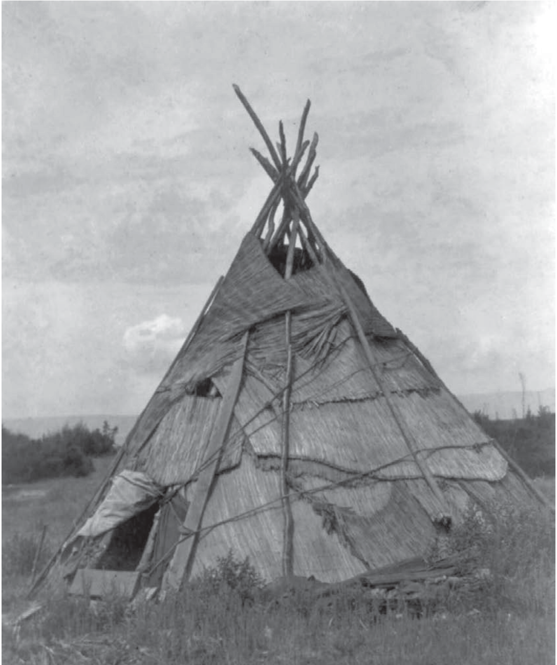
Yakima tepee with reed mat cover, photograph by Edward S. Curtis, c. 1910. Edward S. Curtis Collection/Library of Congress, Washington, D.C. (neg. no. LC-USZ62-99798)
