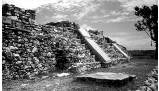
8.7 Examples of Maya stonework: carefully finished facade stones at Copán (top); rougher masonry from Pomoná, Chiapas (bottom).
