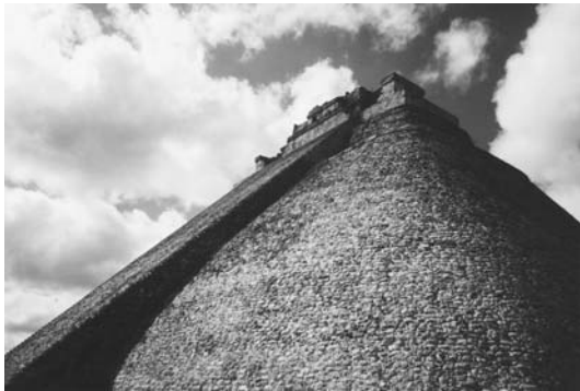
8.1 Pyramid of the Magician, Uxmal. This Terminal Classic pyramid rises 35 meters (115 feet) to the roof on the temple at its summit. The monumentality of the pyramid results from at least four different phases of rebuilding earlier and smaller complexes. (Photo courtesy Lawrence Foster)
