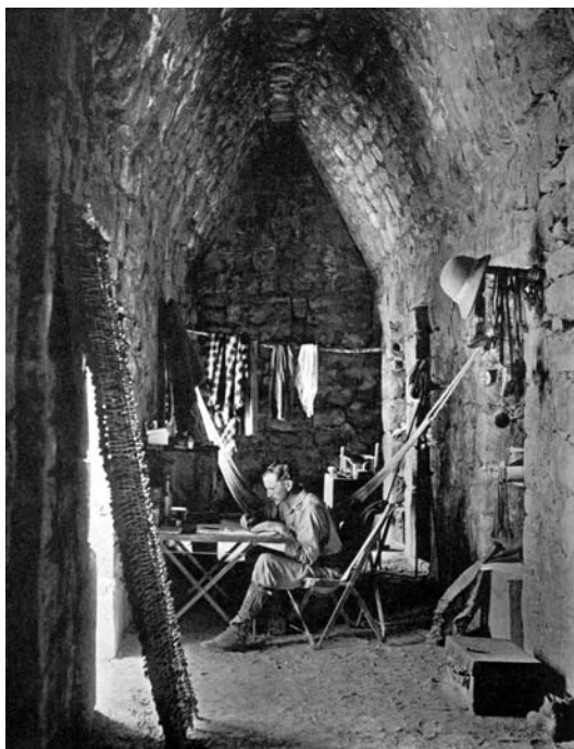
8.3 A corbeled-vault room at Las Monjas, Chichén Itzá, which was used as a camp by Alfred P. Maudslay. (Photo Alfred P. Maudslay 1889–1902)
