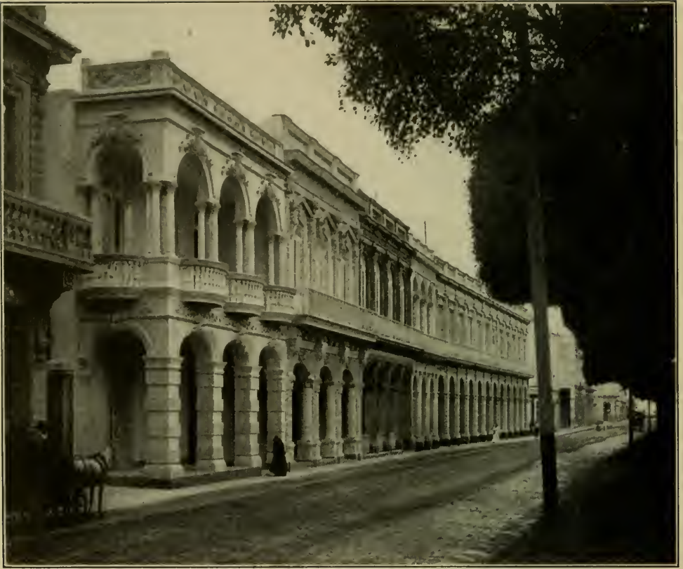
SOME HOUSES ON THE PRADO.
