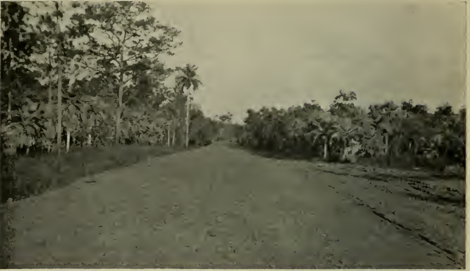
NEW GOVERNMENT ROAD, ISLE OF PINES.
