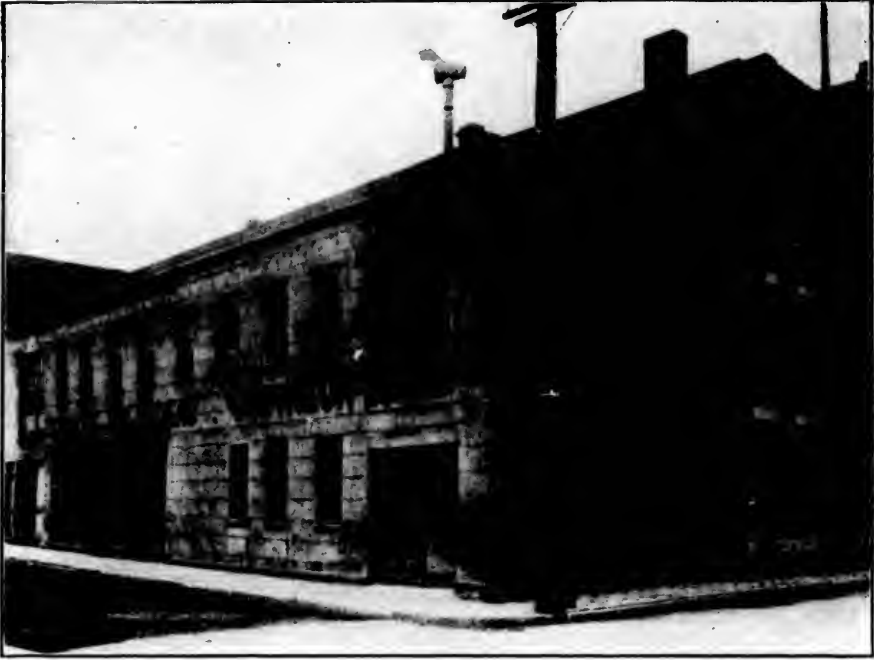
Photo by Harry Richards. Contractor-Roofer
