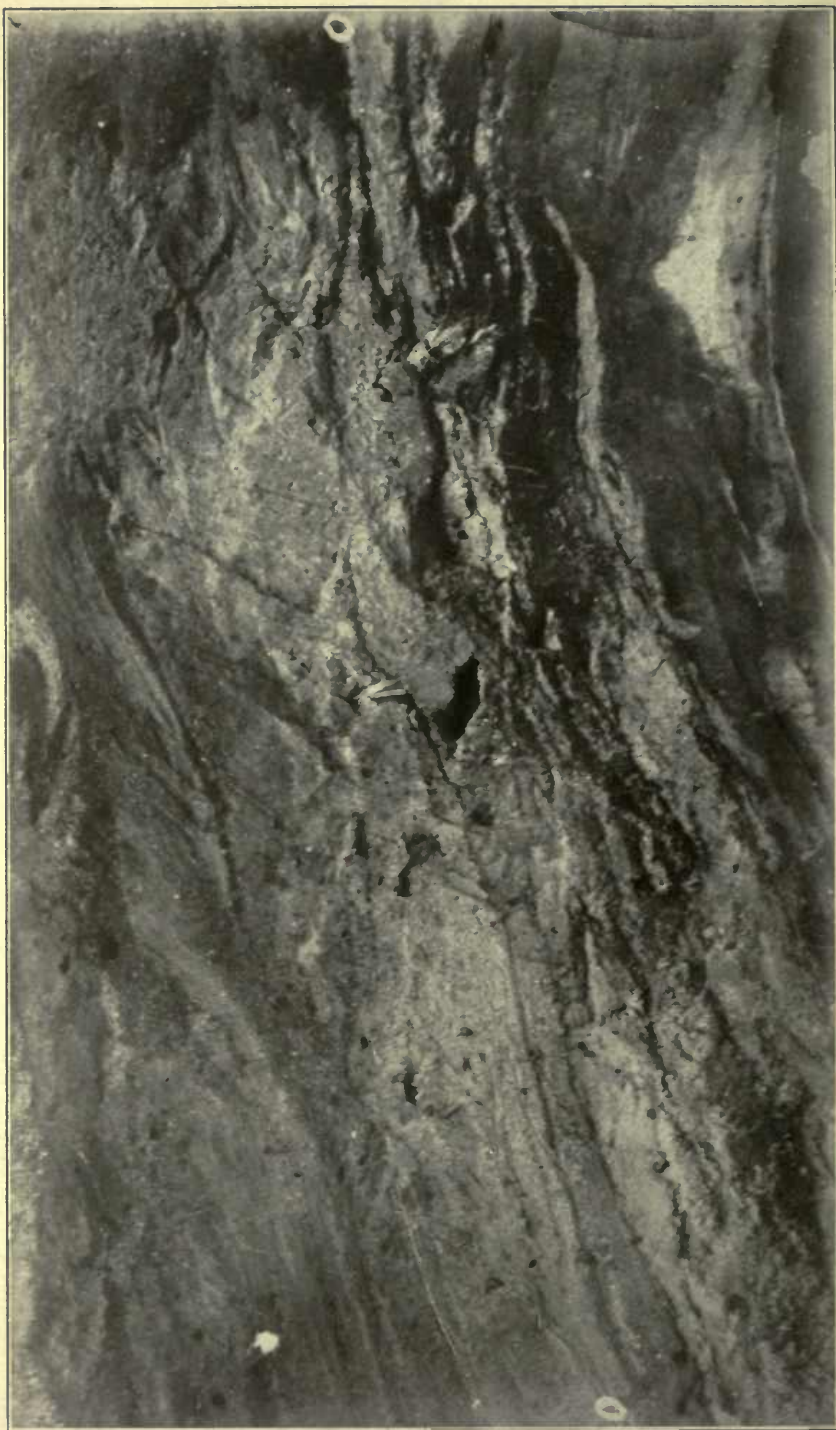
ADVENTITIOUS STRATIFICATION IN THE DUMPS ON THE SOUTHERN BANK OF THE CANAL
