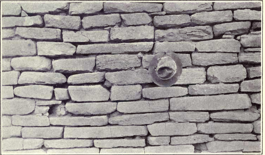
b. MASONRY OF RUIN A
