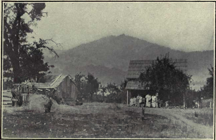
A portion of an orchard may here be seen
