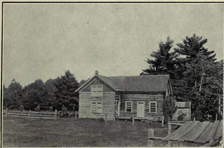
Log-and-plank house of average size
