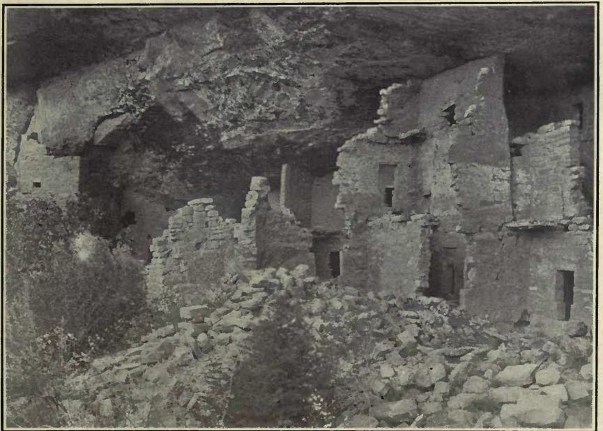
Plaza E, from the south, before repair
