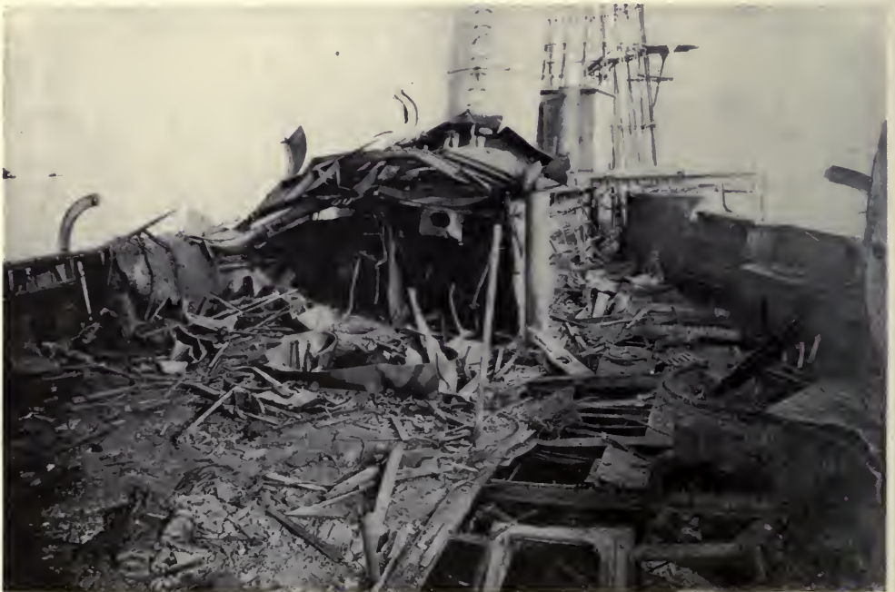
ANOTHER VIEW SHOWING DEMOLITION CAUSED BY THE SAME BOMB (SEE PAGES 340, 343, 347)
