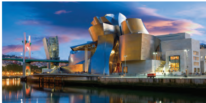
Sheets of twisting titanium cloak the Guggenheim Museum in Bilbao.
