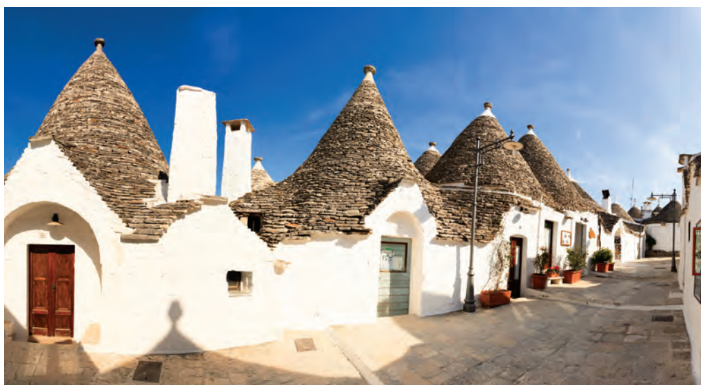
Whitewashed and whimsical, the trulli of Alberobello are built of dry limestone slabs in a style that dates back to prehistory.
