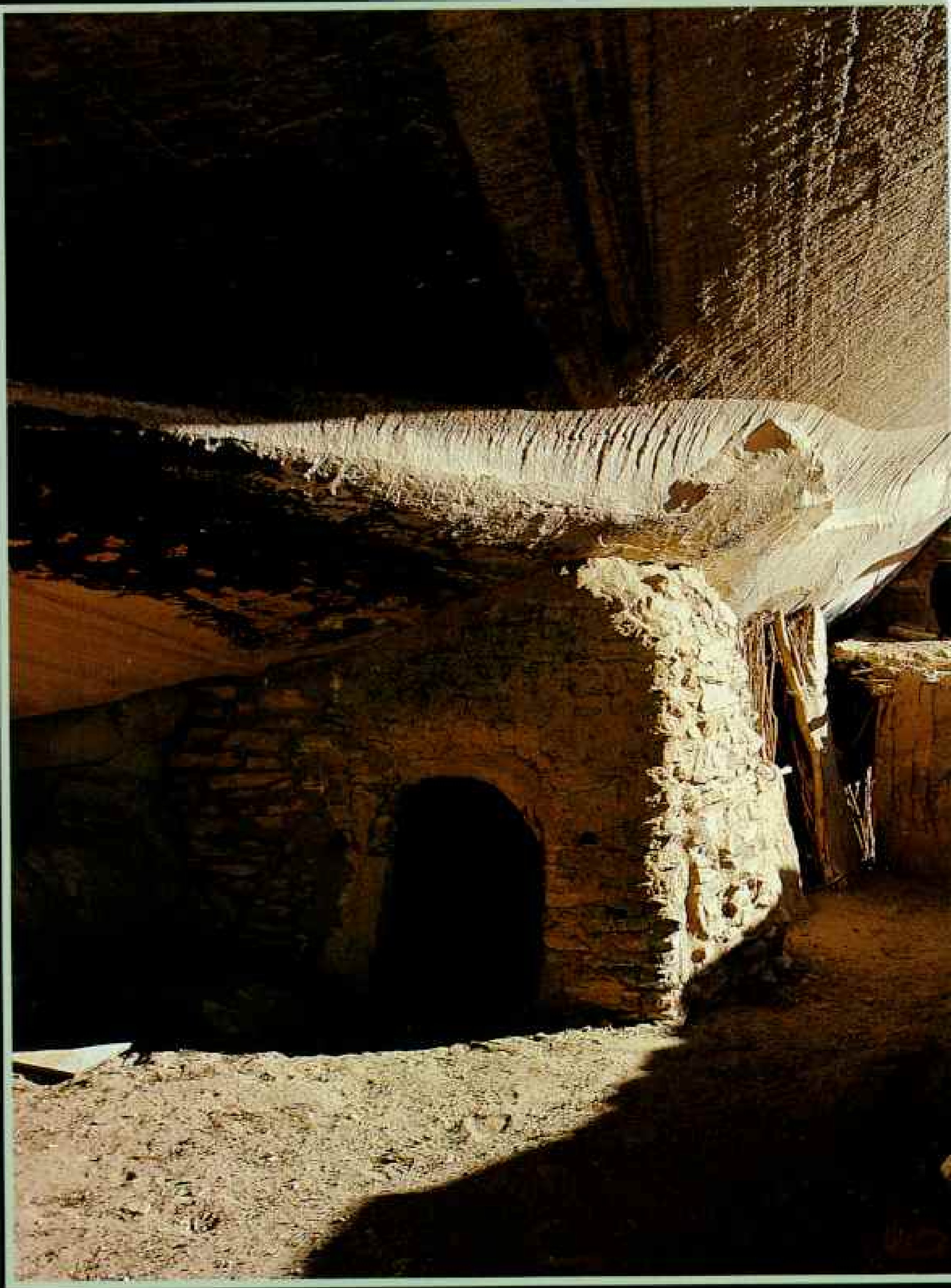
S unbaked mud still clings to the stone walls of Keet Seel, Arizona,
