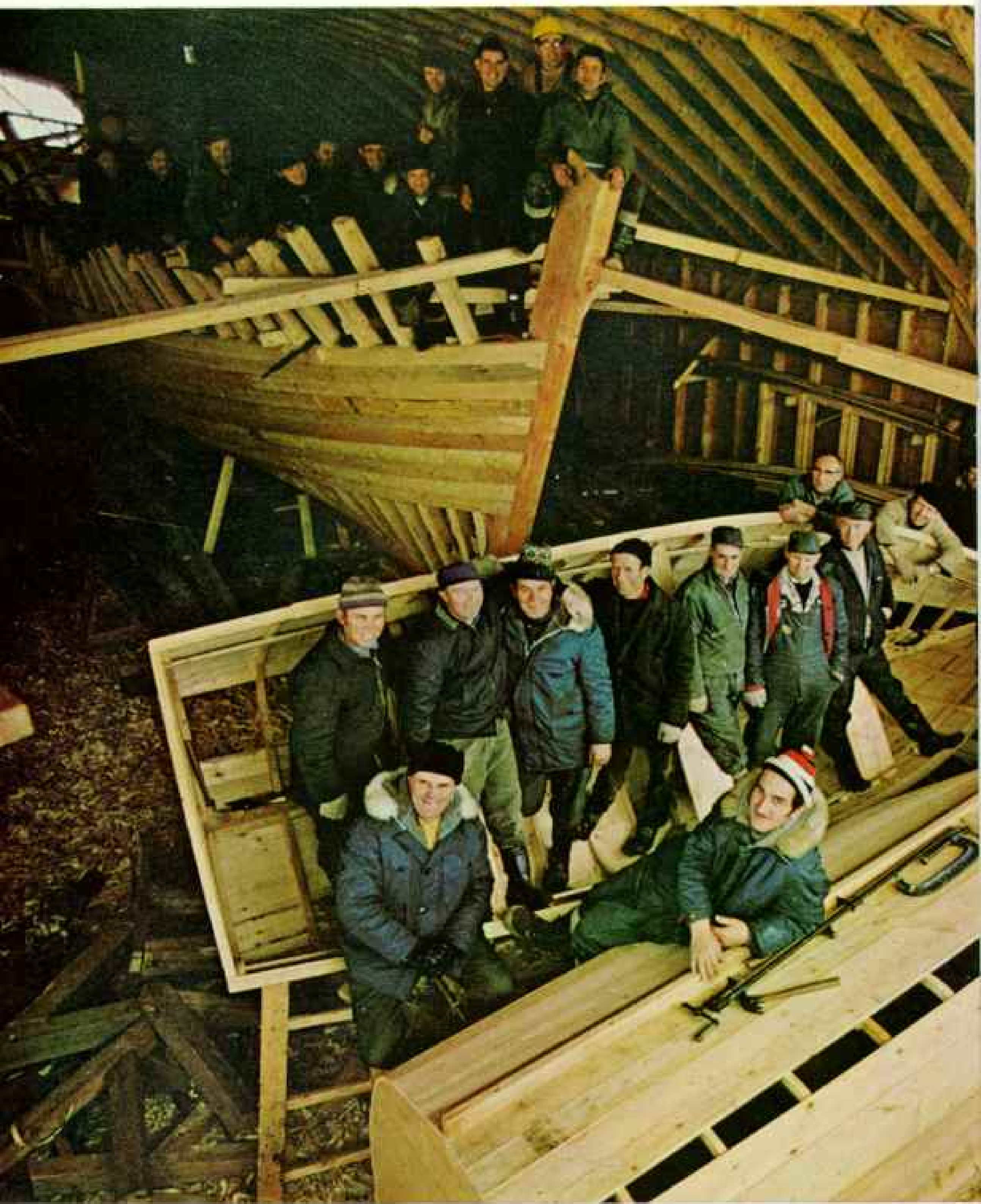
ARCHING RIBS of Newfoundland timber frame the work crew of the Fogo Island Shipbuilding Co-operative. The men perch in smooth-bellied skiffs and the hull of a long-liner fashioned by hand
