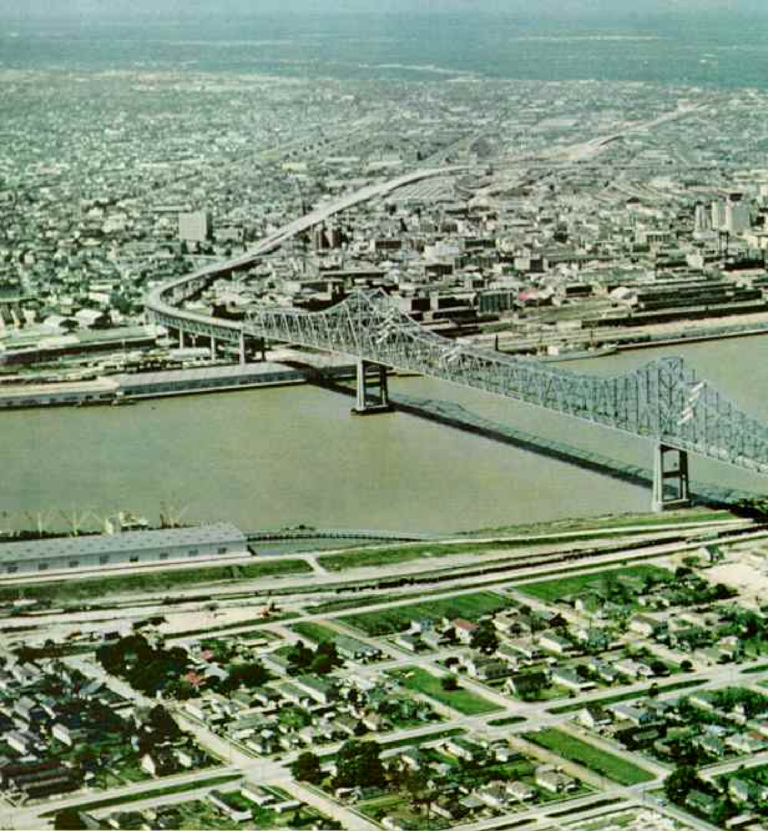
Greater New Orleans Bridge, opened in 1958, clears the Mississippi by 170 feet, linking
