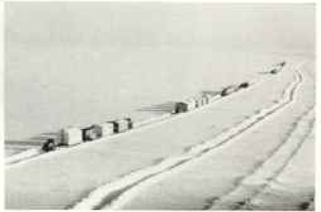
"WANIGANS" ON THE WAY. They're pre-assembled buildings, carried on tractor-drawn sledges.
