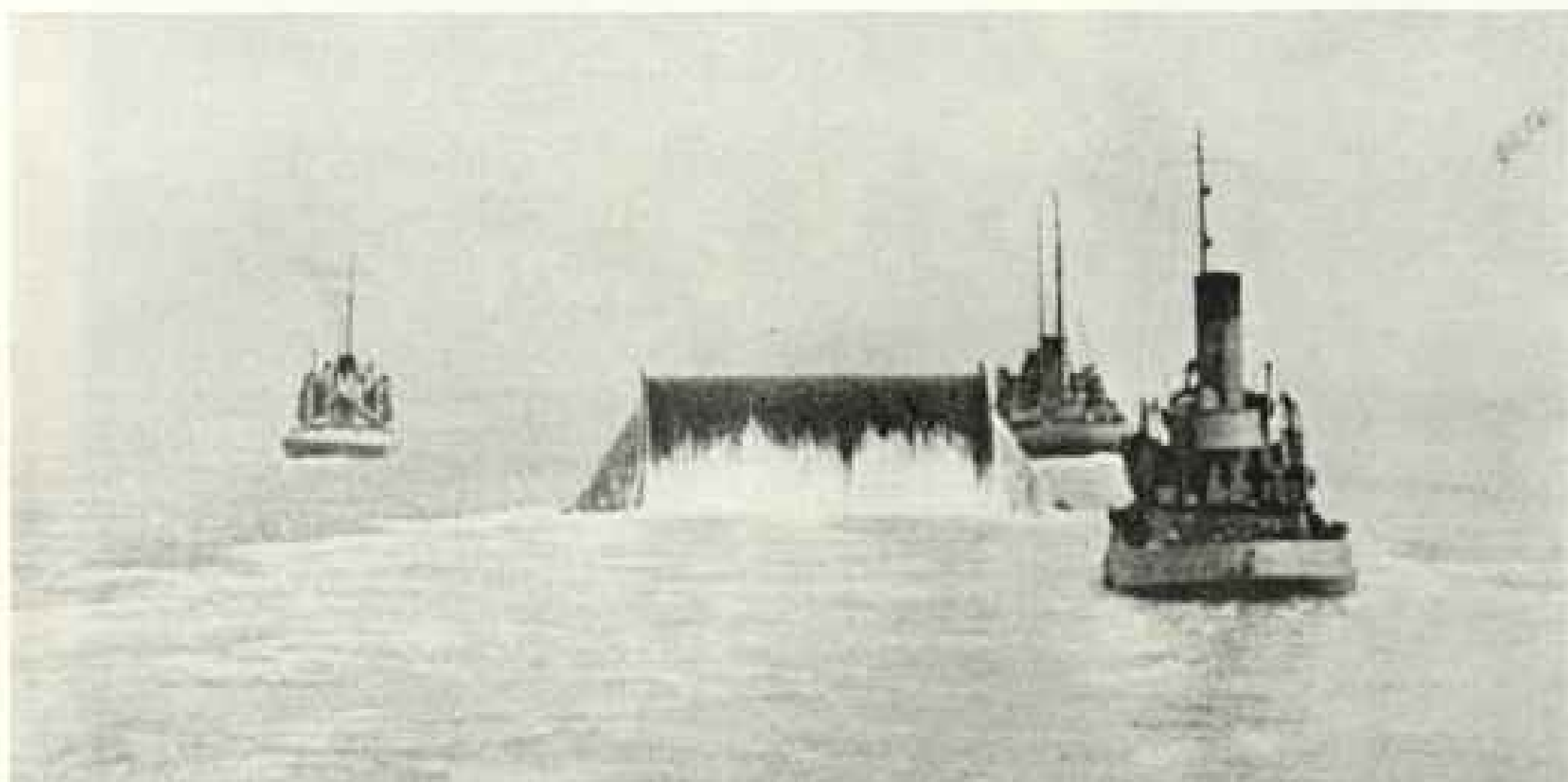
Tugs Tow a Giant Drum, Unwinding Pipe as It Goes, Across the English Channel
