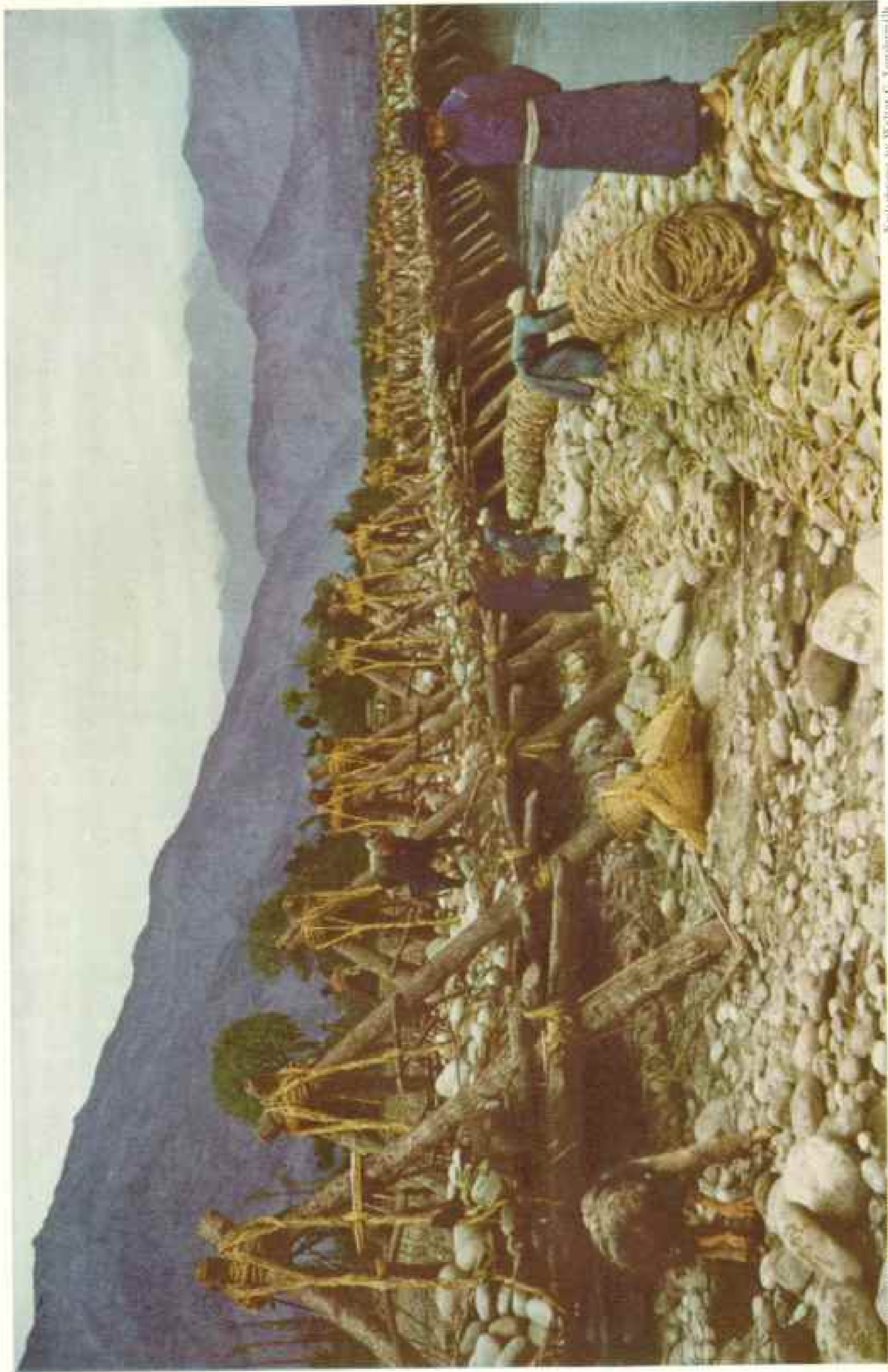
For More Than 2,000 Years These Handmade Headworks of the Tu Kiang Project at Kwanhsien Have Prevented Floods and Famine The men are loading a bamboo "sausage" with stones for use like riprap to bind the stream bank. The heavy timber tripods, bound together with bamboo rope, support a dam filled with stones. To open the floodgates, laborers carry off these rocks and break the contraption apart in the middle by pulling on huge cables.
