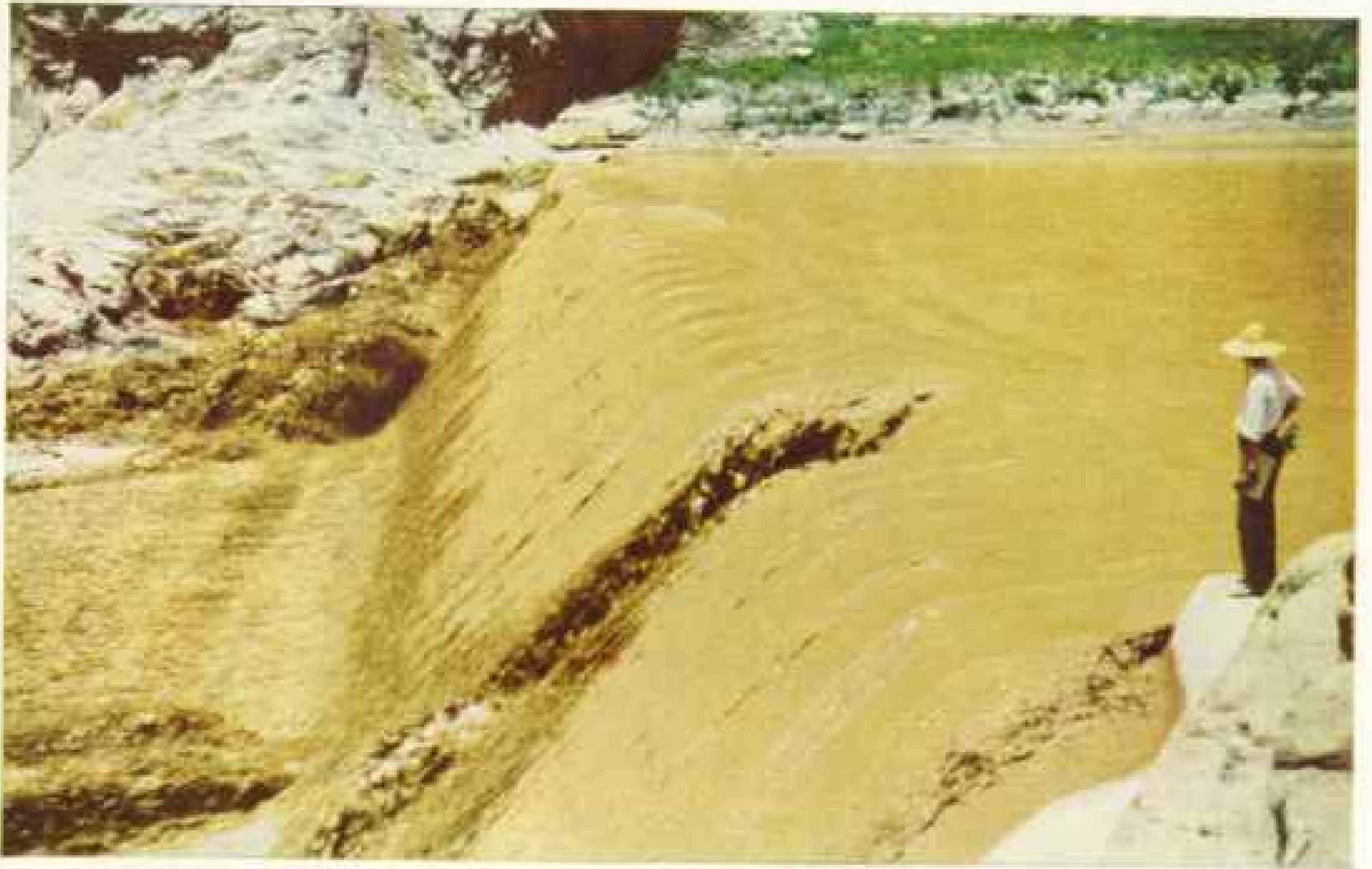
Modern Engineers Have Rejuvenated a King River Irrigation Project Begun 246 n. c. By this diversion dam Li Hsieh and an American, Oliver J. Todd, won the latest round in a 2,000-year battle with silt. The water, the consistency of tomato soup, carries from 25 to 54 per cent mud.
