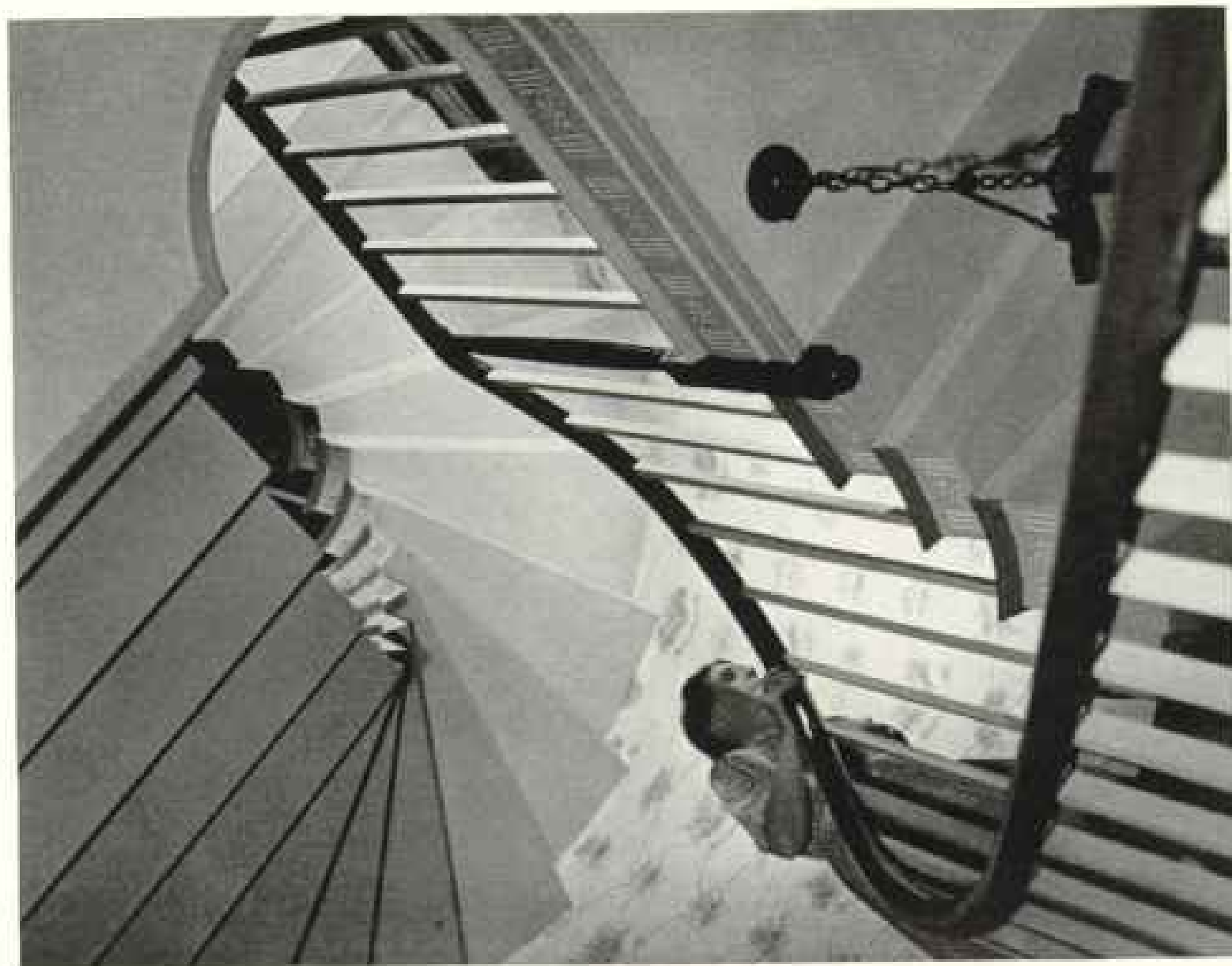
Cobweb of Wood, a "Flying" Staircase Makes a Dizzy Journey for the Eyes
