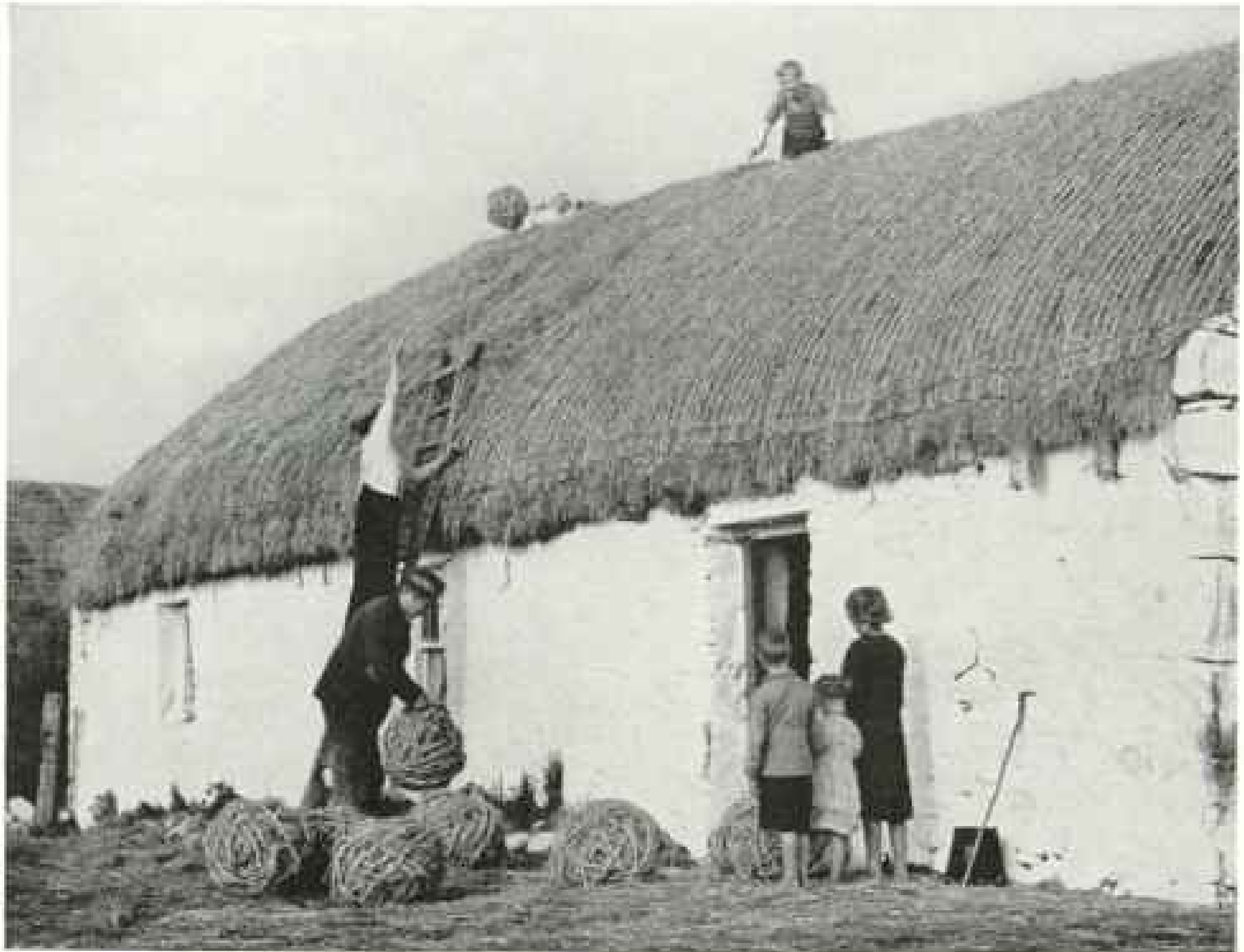
MEN OF THE MULLET TOSS BALLS OF ROPE TO TIE DOWN THEIR ROOFS
