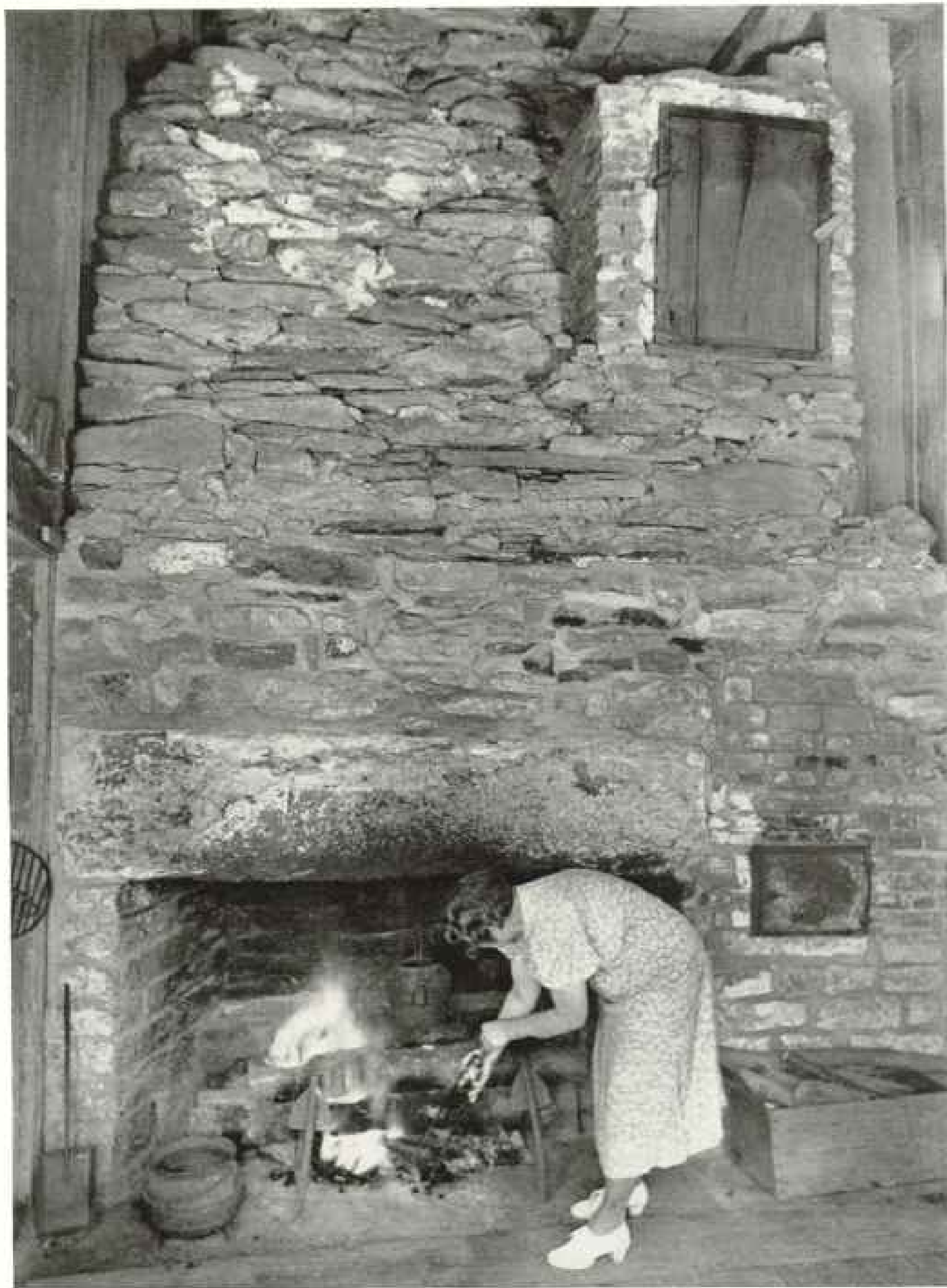
Photograph by Willard R. Culver.
