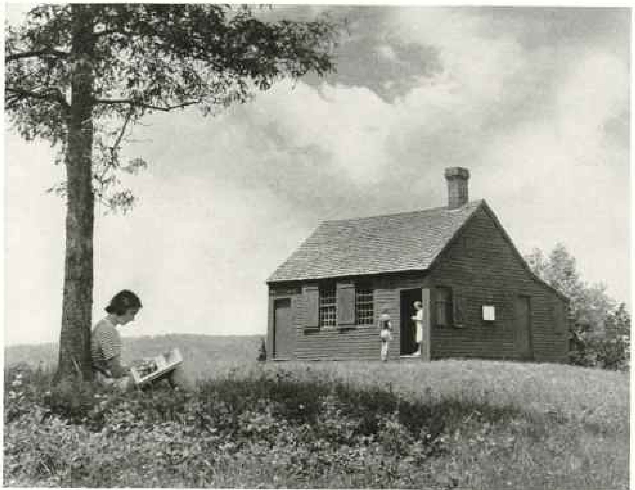
Photograph by Willard R. Culver
