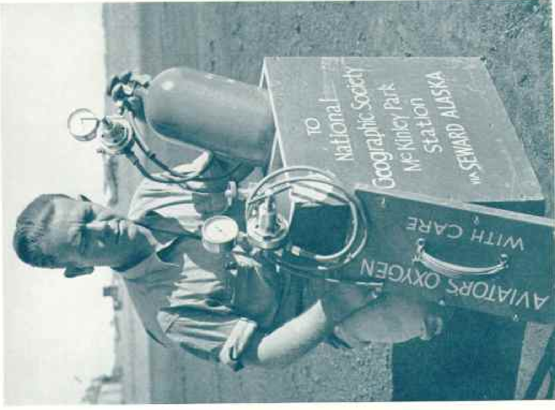
PHOTOGRAPHS BY BRADFORD WASHINGTON "CANNED AIR" FOR FLIGHT IN RARE UPPER ATMOSPHERE A rubber hose conducts the oxygen from cylinder to user's mouth.
