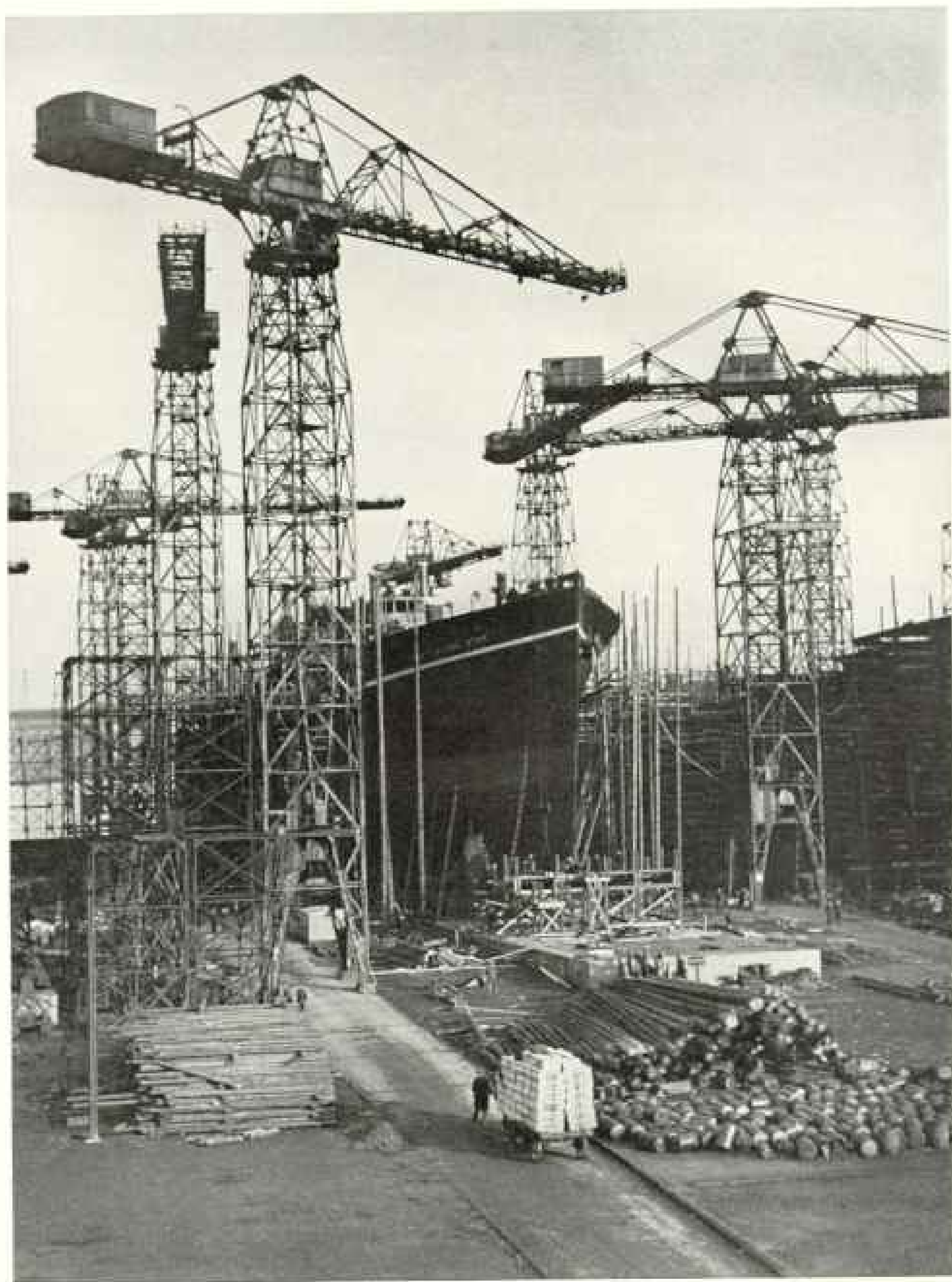
THE "NEW ZEALAND STAR" IS POISED FOR ITS SLIDE DOWN THE WAYS INTO BELFAST HARBOR
