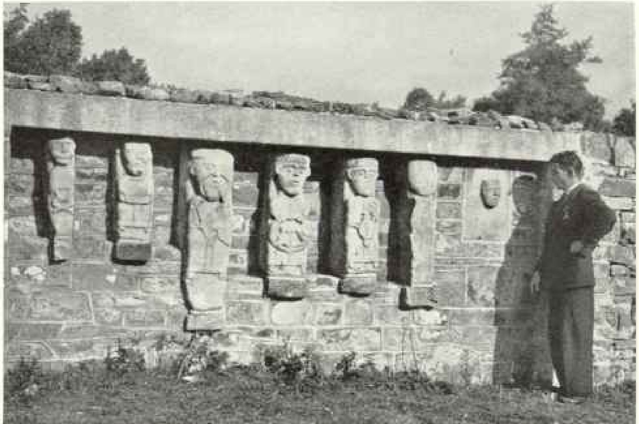
THE MUMMYLIKE CARVINGS ONCE SERVED AS BUILDING STONES IN THE WALL
