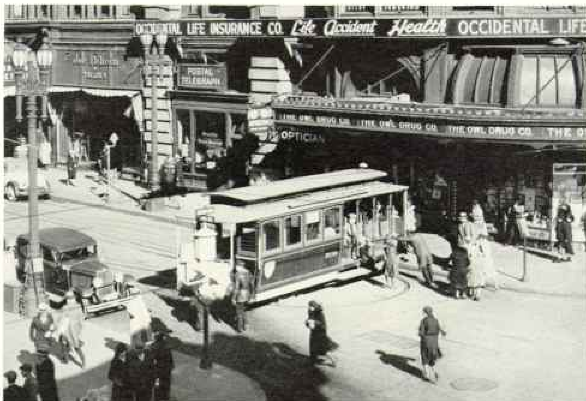
TURNING A CABLE CAR AT THE FOOT OF ONE OF SAN FRANCISCO'S HILLY STREETS.
