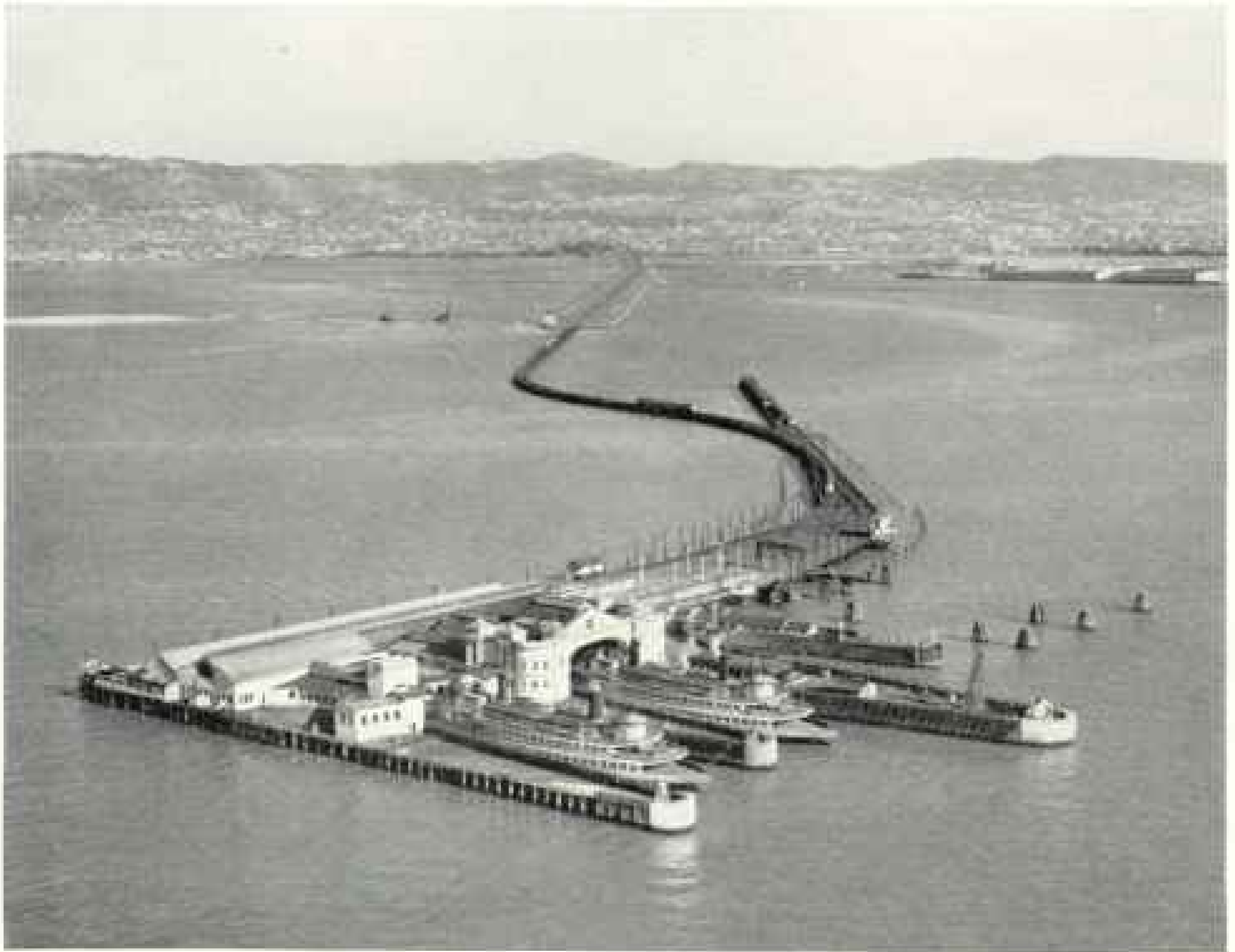
TROLLEY LINES CROSS OAKLAND MUD FLATS TO REACH THIS SLIP, WHERE TRANSBAY FERRIES LOAD AND DISCHARGE
