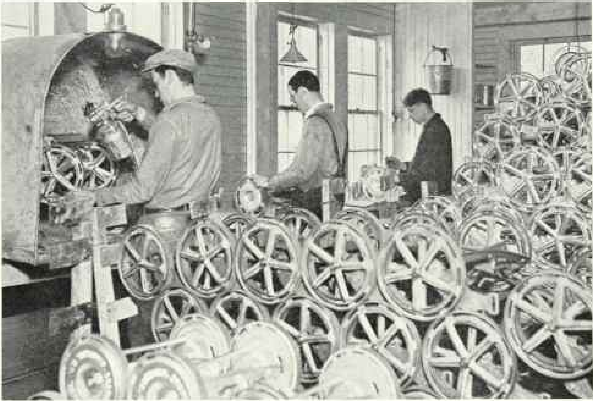
THE SPRAYING BOOTH IN A LAWN-MOWER FACTORY AT HINSDALE
