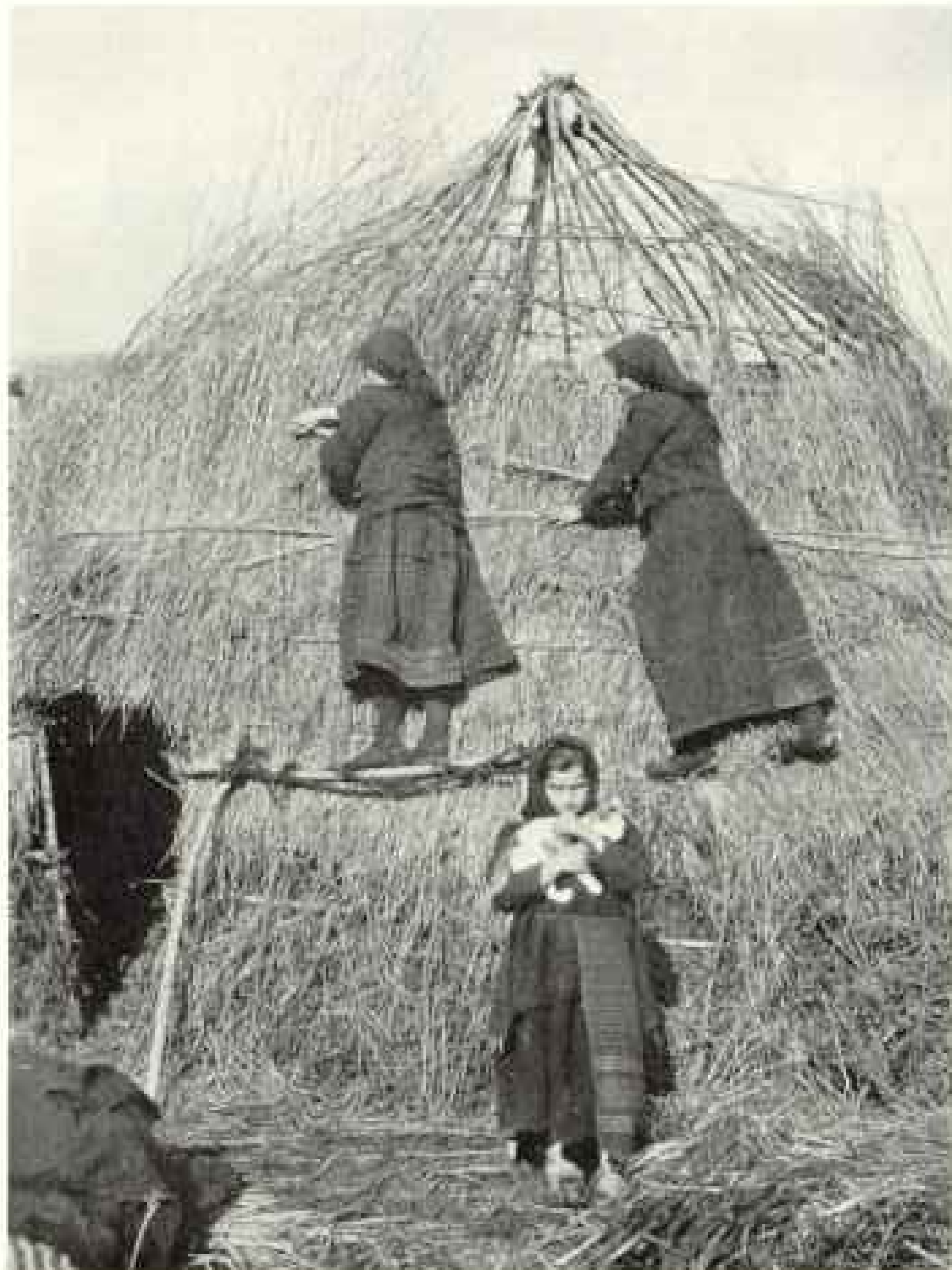
BUILDING A WINTER HUT BESIDE THE IOANNINA ROAD
