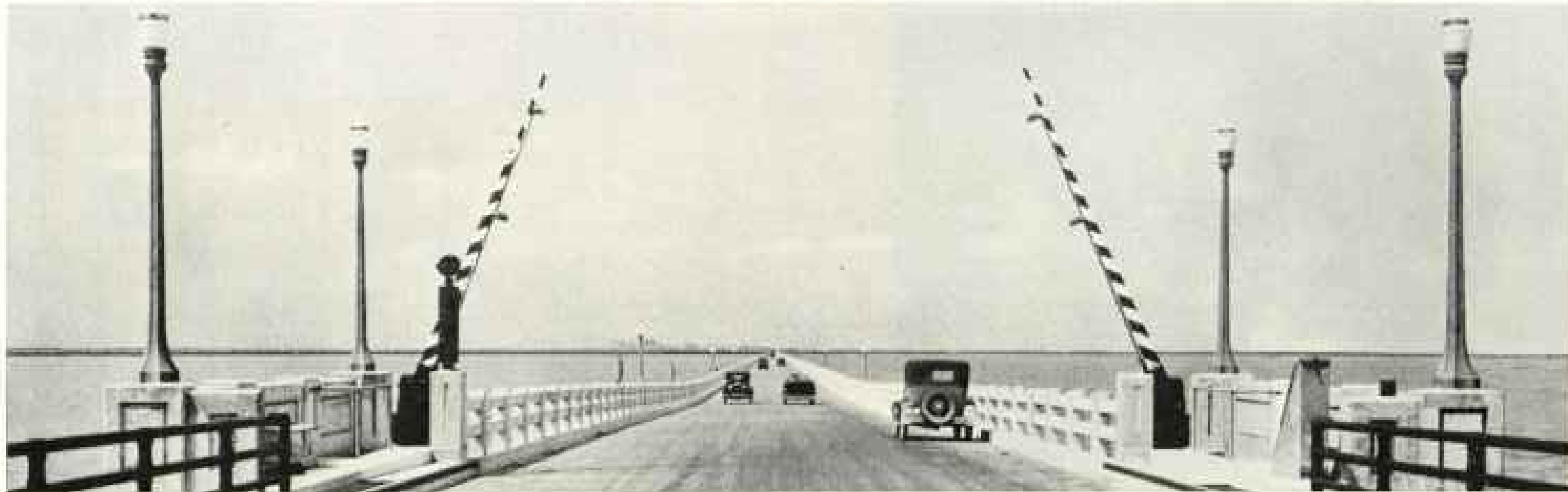
THE CONCRETE TOLL BRIDGE ACROSS LAKE PONTCHARTRAIN IS NEARLY FIVE MILES LONG (SEE, ALSO, ILLUSTRATION, PAGE 482).
