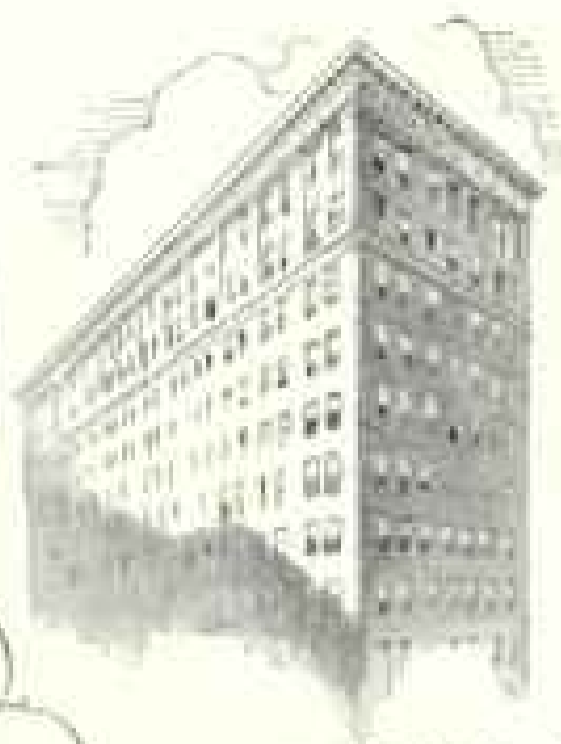
This Office Building at 90 Worth St. is one of many of New York's famous Skyline Te-pe-co equipped.
