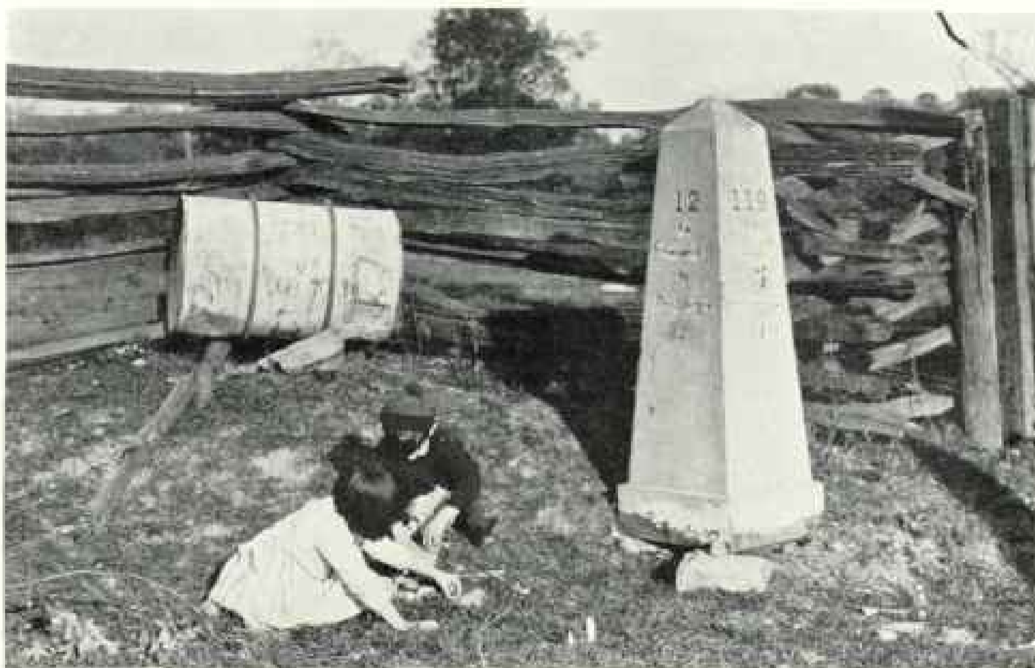
THIS CAST-IRON MILEPOST WAS ERECTED IN THE EARLY DAYS OF THE NATIONAL PIKE
