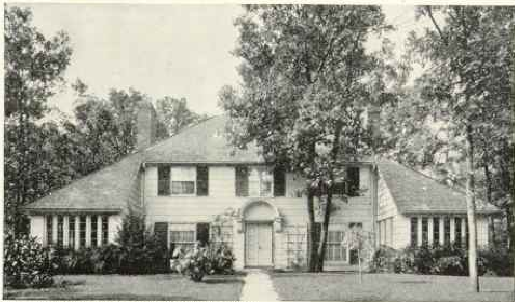
House at Highland Park, Illinois. Robert E. Seyforth, Architect
