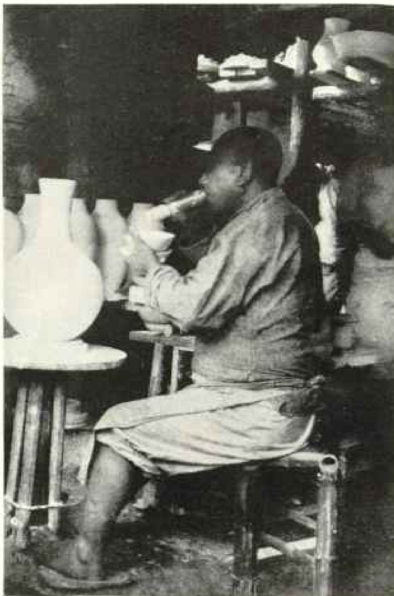
ONE METHOD OF APPLYING PORCELAIN GLAZE
